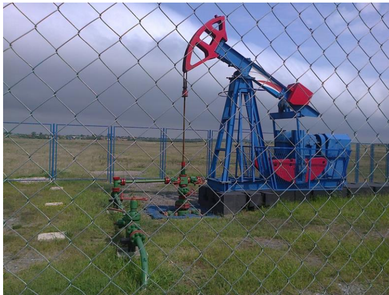
Figure 2. The appearance of the pump well
