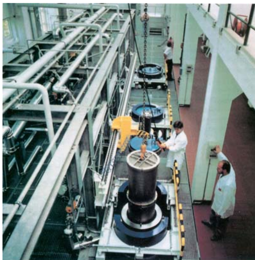
Figure 3. Industrial equipment with 3 extractors (500L each), 2 separators (375L each) and 1 separator with 175L. Extraction pressure 440 bar (UHDE) [12].
